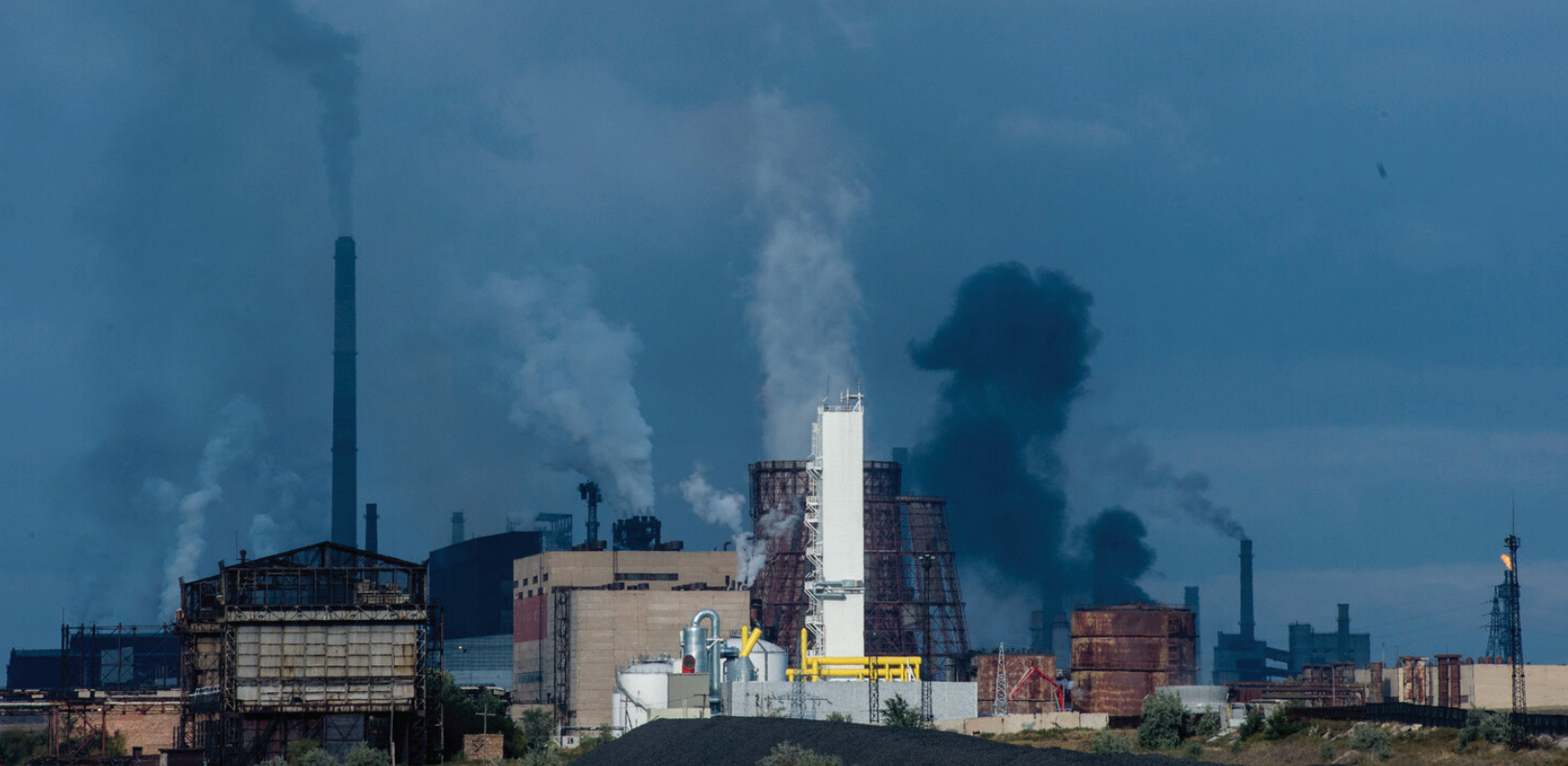
A Steel Mill in Termitau, Kazakhstan (photo by ADB).
